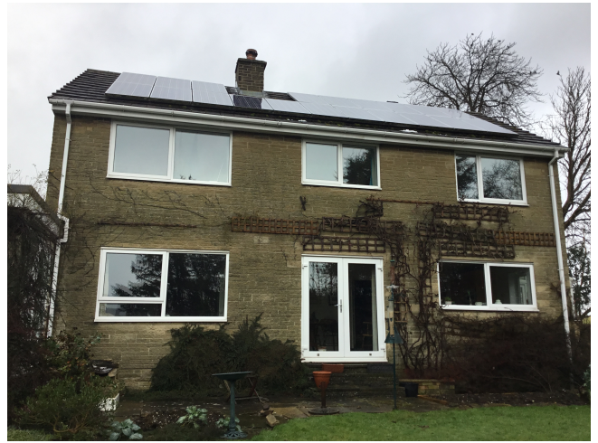
South elevation showing solar panels on south facing roof
