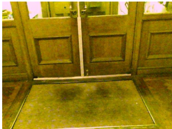
Draught exclusion - Completed
